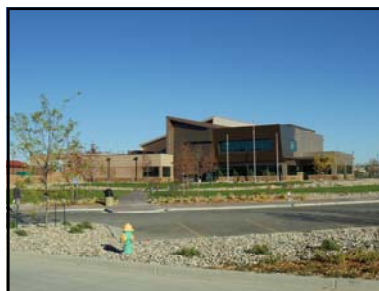
National Guard Readiness Center Grand Junction, CO
