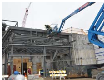
ACWA Plant Construction
